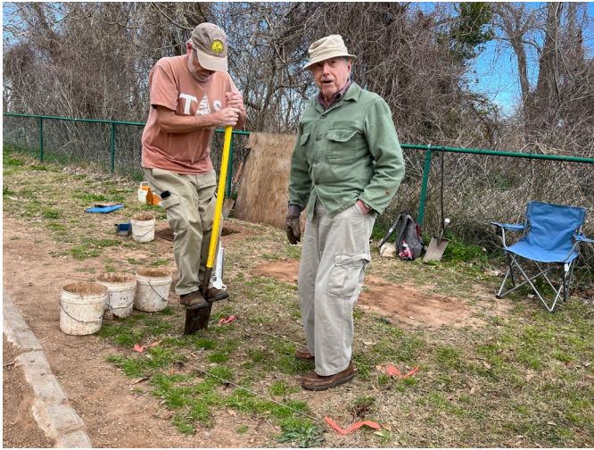
Bruce Grethen and Bob Crosser are breaking ground on a new 2'x4' pit at our excavation site.
